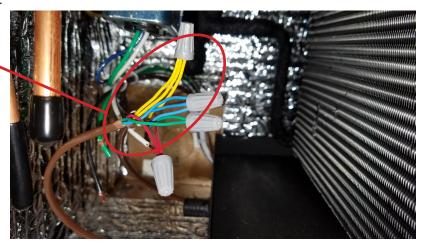
Condensing Unit: Connect the other end of the 18-2 low-voltage thermostat wire to the grey and purple wires located in the grey electrical box on the condenser skid.
