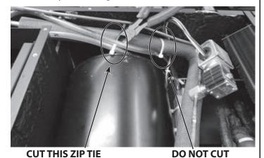
8. Pull tubing out of housing to allow room for brazing. Make sure tubing protrudes out of the housing and the drain line is moved out of the way as shown.
