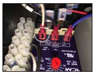
Using the closed end terminal crimp the #1 wire with the remaining low pressure switch wire.
