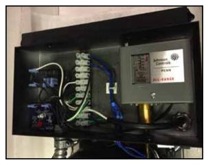
Secure both wires into the H1 lever connector.
