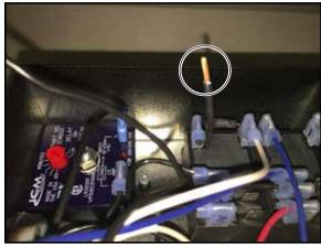
Secure the bare end of the wire from the #1 terminal on the Delay on Break timer inside of the C lever connector.
