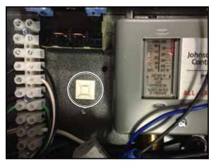
Remove the adhesive backing from the bypass timer.
