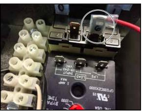
Zip tie one of the high pressure switch wires and low pressure switch wires together.
