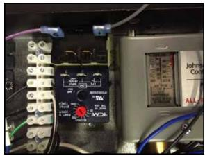
Route the #10 wire with the blue disconnect labeled **T** down through the cord squeeze.
