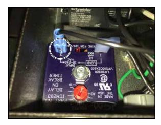
Cut the blue disconnect off the wire that was connected to the #3 terminal of the Delay on Break Timer. Strip the end of the wire to a length of 3/8".
