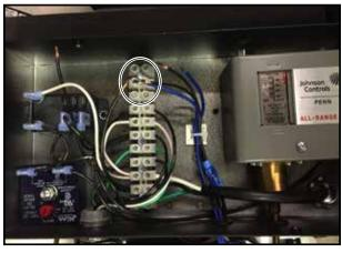
Cut the zip tie holding the high and low pressure wires.
