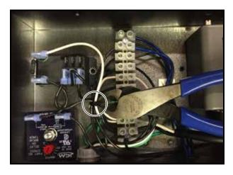
Using a flat head screw driver loosen the six terminal screws outlined in red, and remove the wires from the terminals.
