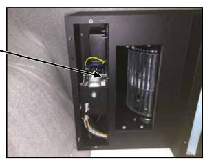
Re-install the electrical panel using the 2 Phillips head screws removed in step #7.
