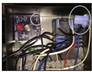
Crimp the blue disconnect labeled 3 onto the loose wire coming from the Johnson control. (It was disconnected from the terminal block in step 16)
