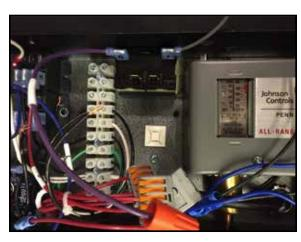
Using a flat head screw driver remove the cable tie holder.
