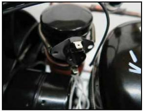
Secure the blue female disconnect labeled **T** onto the bottom terminal of the thermal switch.
