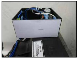
Using a step bit, drill a 5/8" hole through the cross. (Be sure not to drill into the electrical components.)
