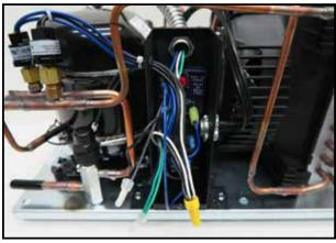
Remove the yellow wire nut from the 4 neutral wires.
