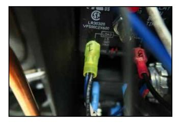
Zip tie wires **7**, **10**, **11** & **12** from the Cold Weather Start Kit box to the fan shroud as shown.
