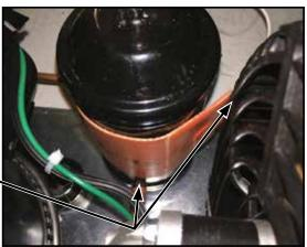
Place the other silicone heater on the receiver in the location shown. The heater will not adhere completely, there are hose clamps installed later in these instructions that will keep them firmly in place.
