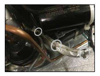
Slide the heat shield over the wires up to the condenser fan motor and zip tie to capacitor bracket as shown.
