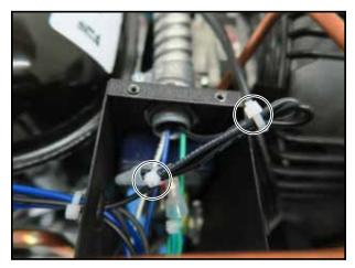
Remove the yellow female disconnect from the #8 terminal on the contactor.
