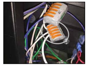
Secure one of the thermostat wires and the yellow wire from the transformer into a lever connector.
