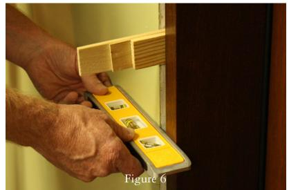
• Check that the jamb is flush with the surface of the drywall on both sides oft the jamb. [Figure 6]
