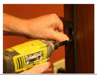
• Secure the strike-side of the jamb under the weather stripping at the top and bottom of the jamb at hinge heights with 2" screws. [Figure 10]
