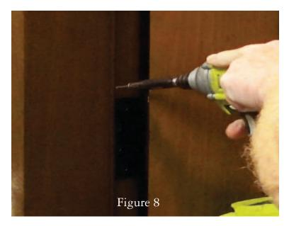
• Now move to the strike-side jamb. Remove the lock set strike plate from the jamb, drill a pilot hole inside the strike mortise and away from the strike and screw holes. Drive a 2" screw through the jamb and into the framing. Close the door and check all gaps. If adjustment is needed, remove a 2" screw, adjust hinges and reset the screw. [Figure 9]
